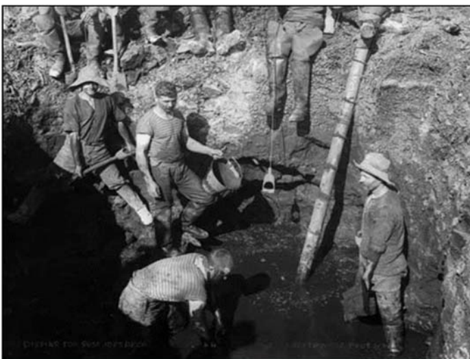
Gum diggers often worked on the drier hills in winter and headed for the swamps in summer. Teams would locate the gum using very long spears (centre). Here they are keeping the pit relatively dry with a simple hand-powered water pump as men took turns to dig. Photo source: lpenz.org.nz
